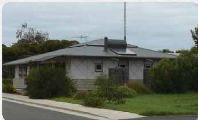
Ceduna disability support accommodation
